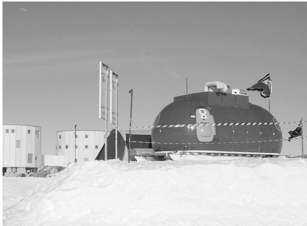
Figure 1: The AASTINO installed in front of Concordia station.
