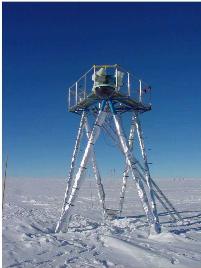
Fig. 4. The 7.5m high G-Tower supporting a 500kg low-power telescope mount at South Pole Station.
