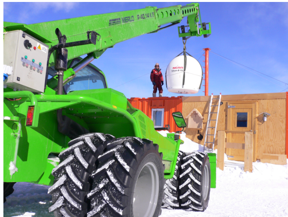
Fig. 2. A satellite communication dish is lifted onto the roof at Dome C. Infrastructure already in place at South Pole and Dome C is well suited for the construction of astronomical facilities.
