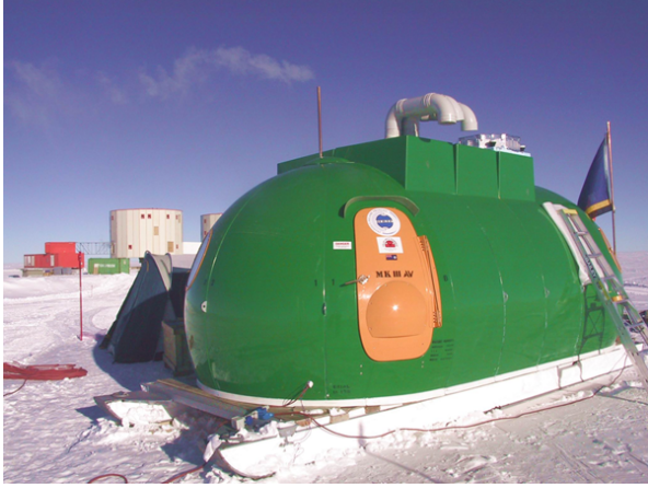
Fig. 3. The AASTINO is a robotic site-testing observatory that can operate completely unattended.
